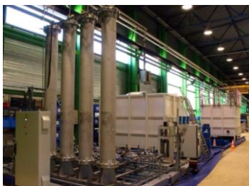
ODySEA demonstrator on the premises of Cetim, Nantes (complete installation)
